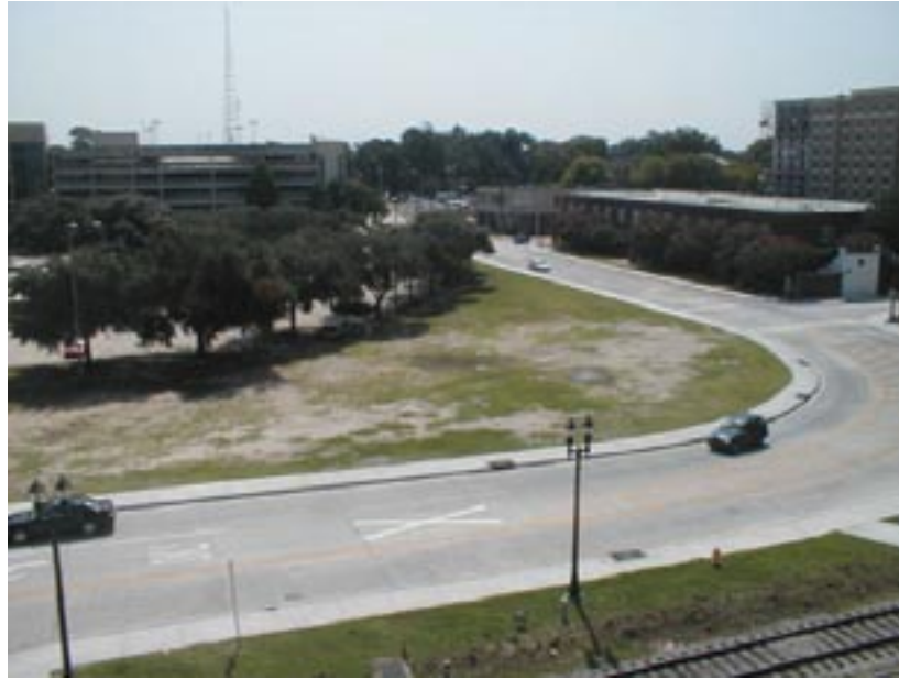
River Road Realignment - Completed May 2002
